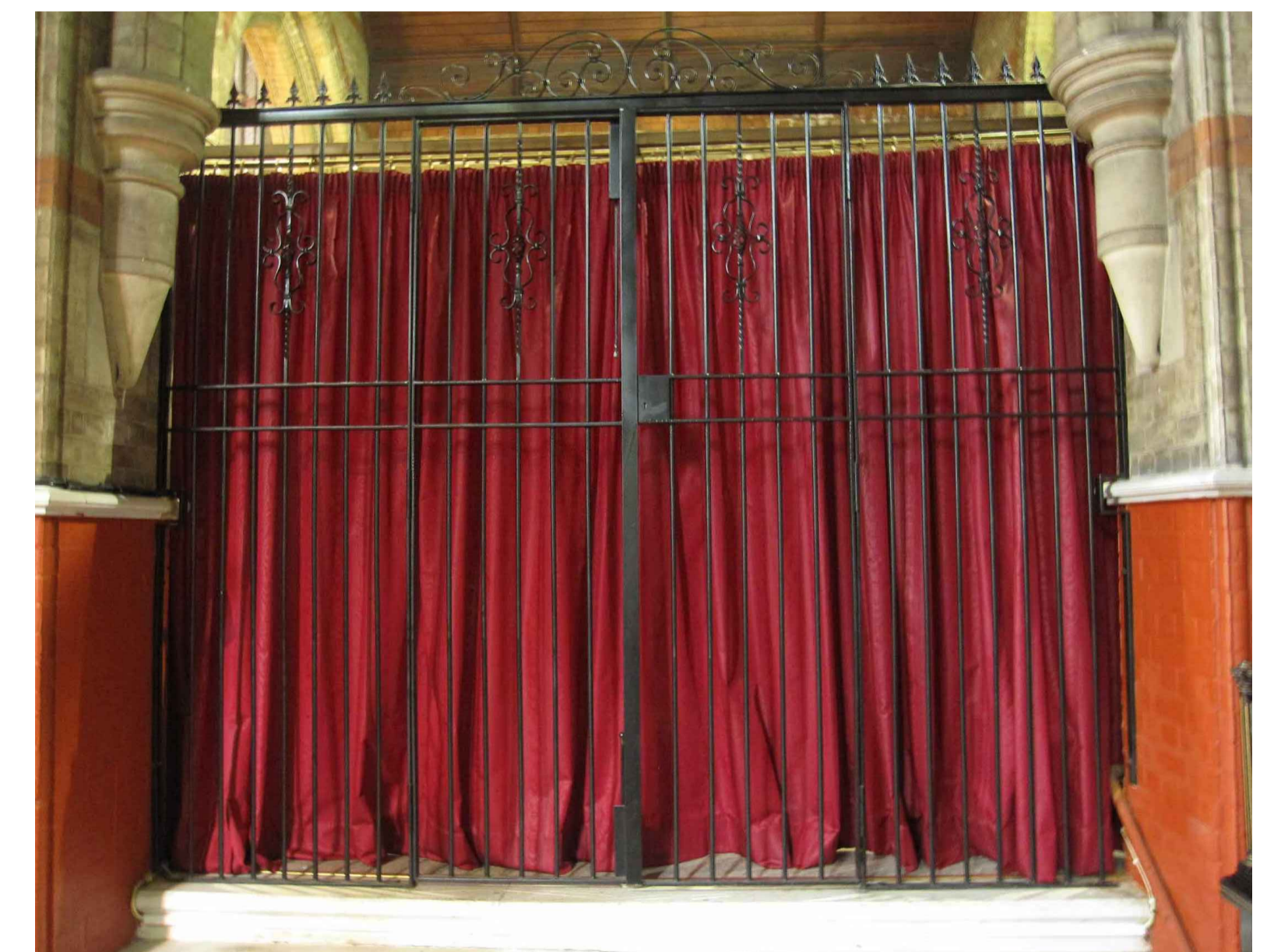
04 Existing Railings and Gates to Vestry NTS
